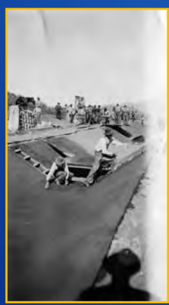
Concrete canal lining project, 1913
